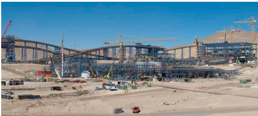
Leaving aside expansions, Peru does not have any new large projects under construction right now. Photo courtesy of HV Contratistas.
