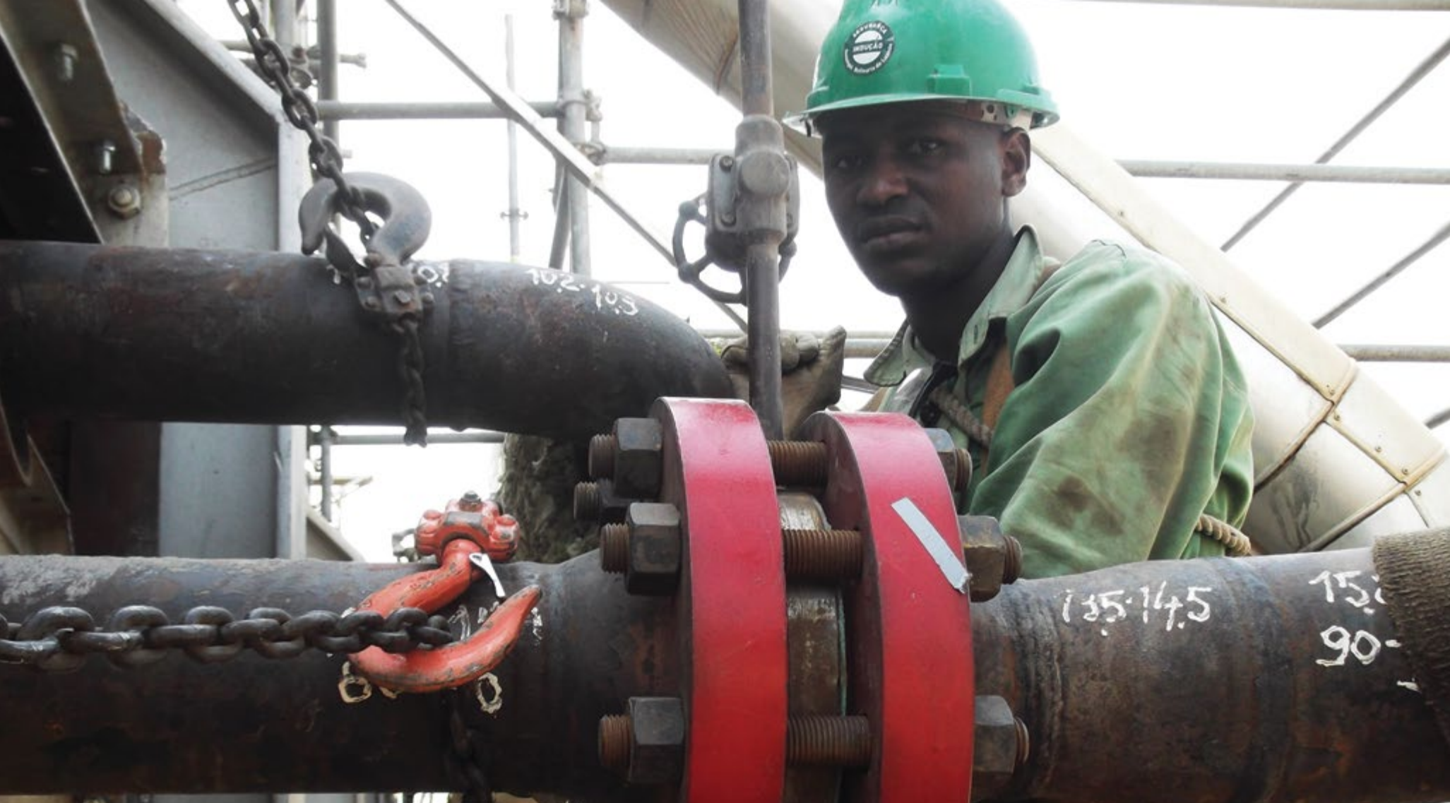
Image: PROMETIM performing a hydrostatic high pressure test at Luanda Refinery in Angola.
