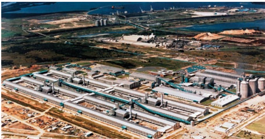
Mozal Aluminium Smelter Alumina Handling, Mozambique. The scope of work comprised the supply, fabrication, corrosion, protection, transport and erection of structural steelwork, platework and piping installation. Photo courtesy of Group Five.
