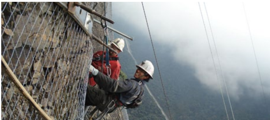
High scaling crew installs screen mesh and bolts on HEAT (Heavy Equipment Access Trail) 2.1km area. Photo courtesy of Redpath.
