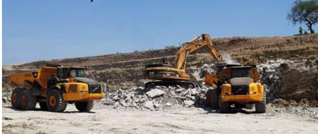
Overburden removal. Photo courtesy of PW Nigeria.
