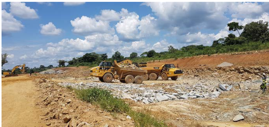
Construction of 1km power canal at Kibali. Photo courtesy of IOB.
