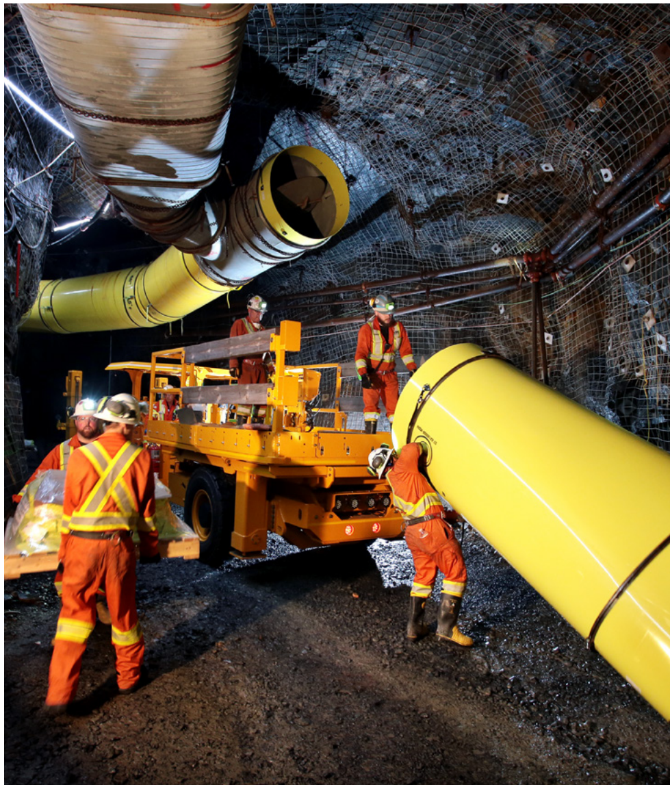
Image courtesy of DSI Underground
