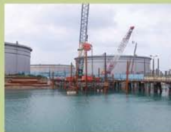
Marine Piling for Refinery Modification Works
