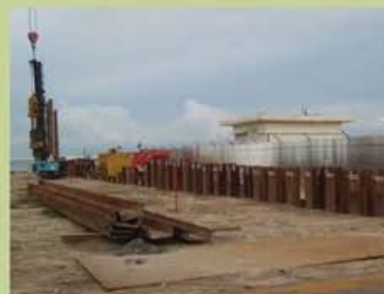
Construction of Cofferdam for Subsea Pipeline Works
